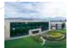
The New Factory
