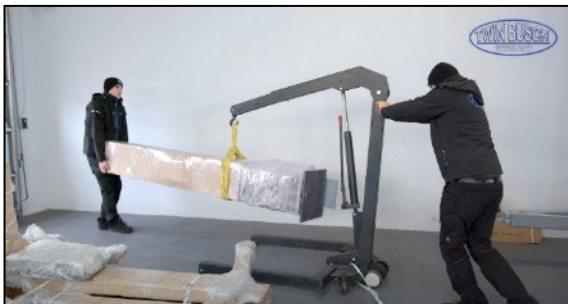
Illustration: Lifting the column
