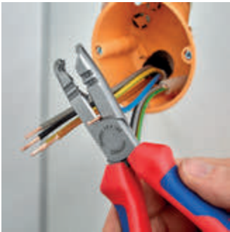
Cutting when shortening single conductors
